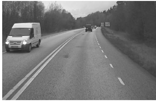
Various street surfaces
